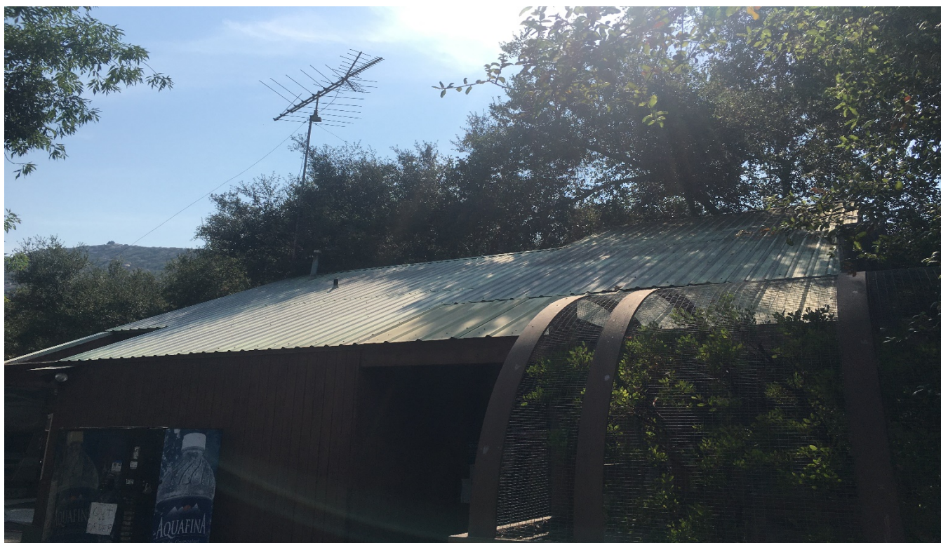
Photo 1: Picture of metal roof with penetrations.
